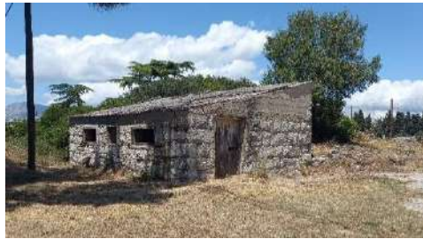
Figure 28. Auxiliary building 1 (Storage – cadastral parcel no. 7372) for storing tools, etc.
