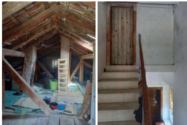
Figure 22. The attic of the Building 2A
